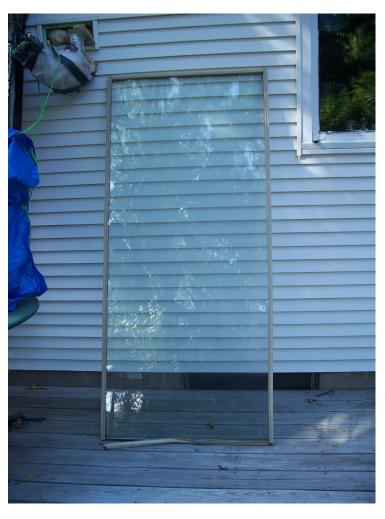
Obviously here I've taken the wood off from around the glass. The glass measured 76 1/4" x 34 1/8" x 6/8 so it's quite a bit bigger then the original. In fact you can see in this picture it's almost as tall as the original, and the old one is sitting on a table!
